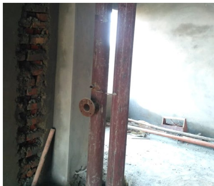
Fire Protection system
