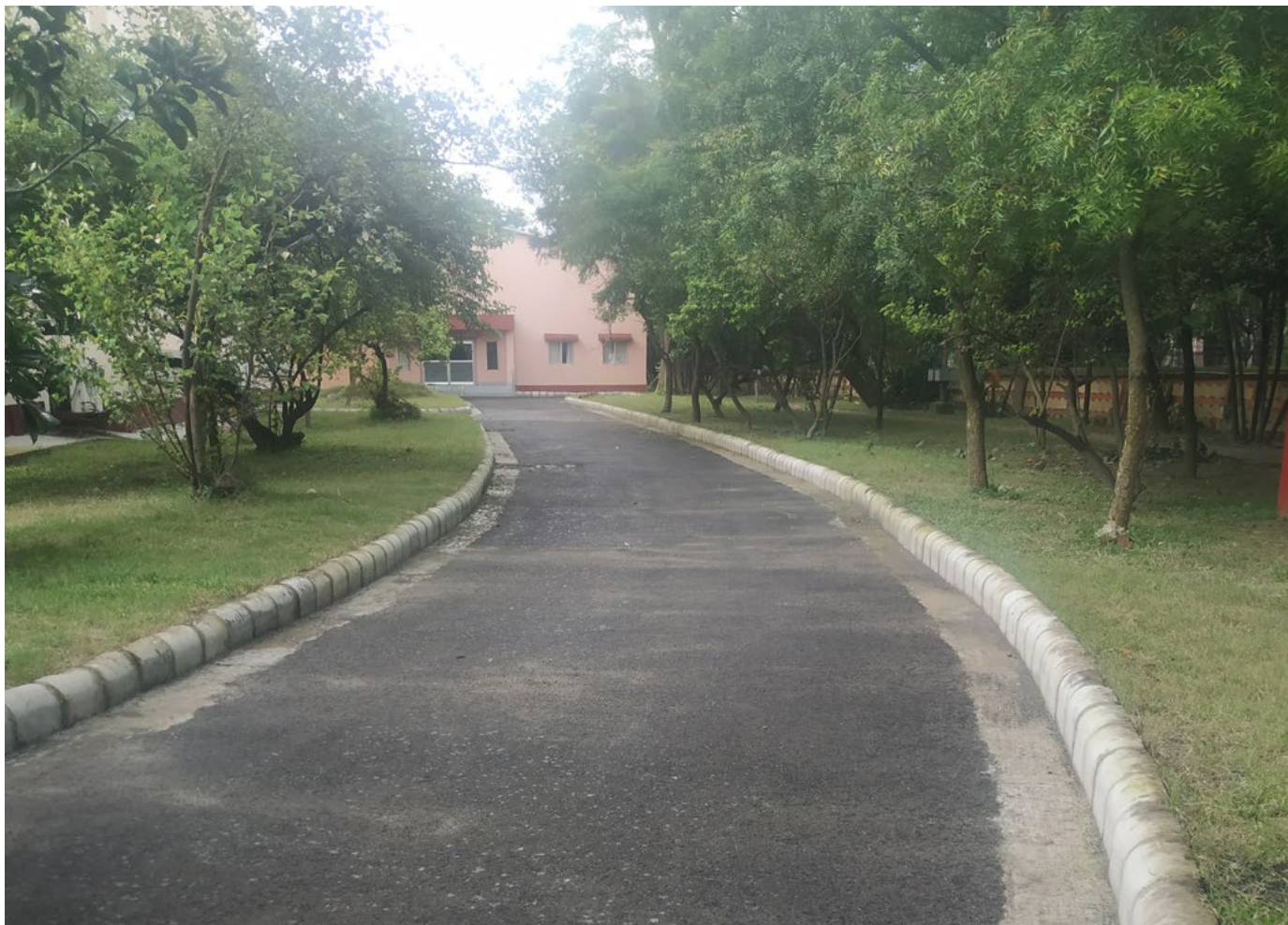
New Road Constructed From Main Gate to Lab II
