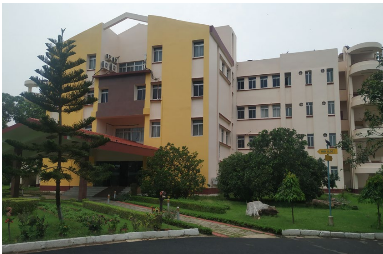
Exterior Painting Main Building
