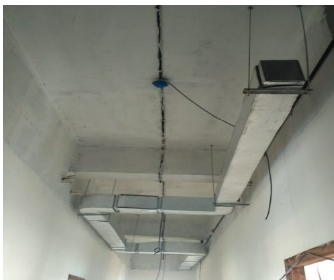
VRF AC Works
