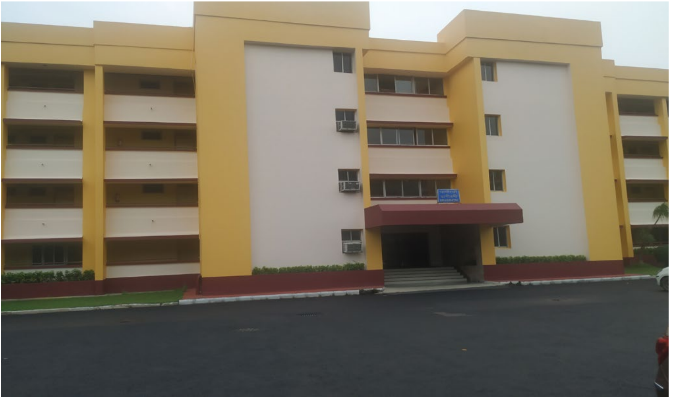
Exterior Painting Bhagirathi Building
